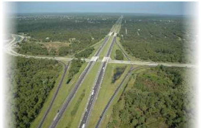
Sumter Boulevard Interchange
