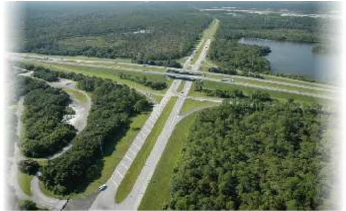
North River Road Interchange
